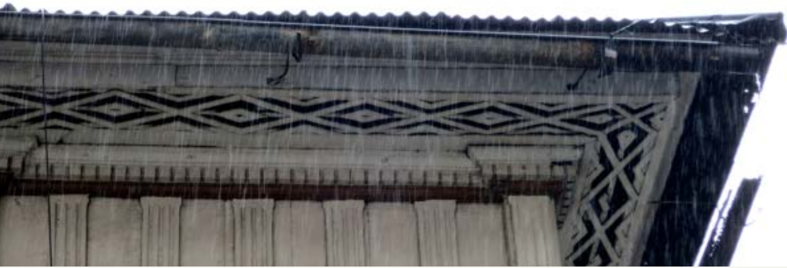
Detail of roof eaves, Photo Credit: Roz Li
